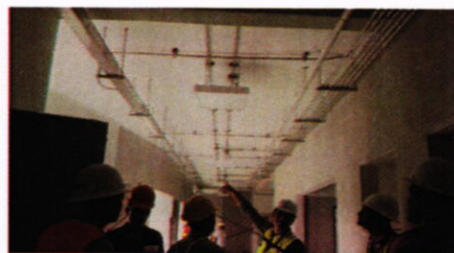
Fachada interior pasillo frontal, CURLP
