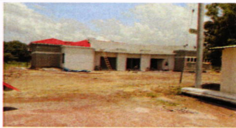
Fachada frontal, CURLP
