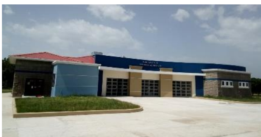
Vista fachada principal
